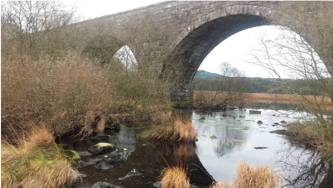
Figure 63: Start of survey at the bottom of Stroan Loch (NX 264701 569972)
