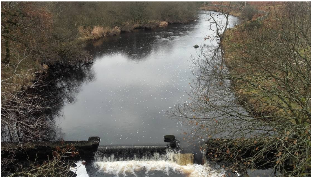
Figure 78: Hensol Weir located at NX 266364 570073, glide habitat was recorded upstream. The impact of this weir on fish migration and sediment transport should be investigated
