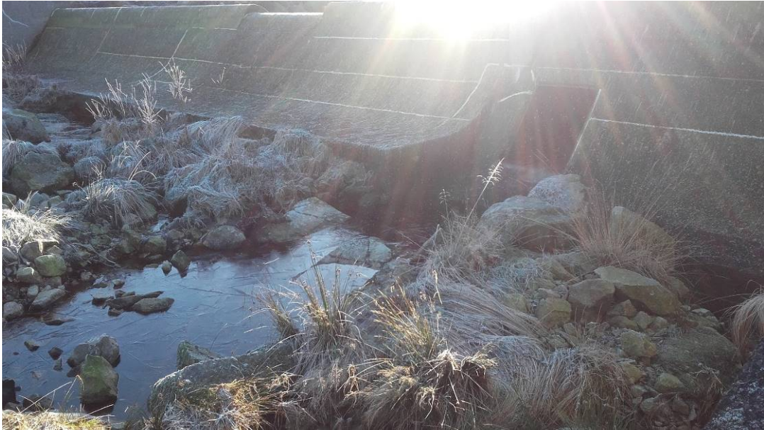
Figure 1: Downstream of dam at Pullaugh Burn, start point for habitat survey (NX 254418 574123)
