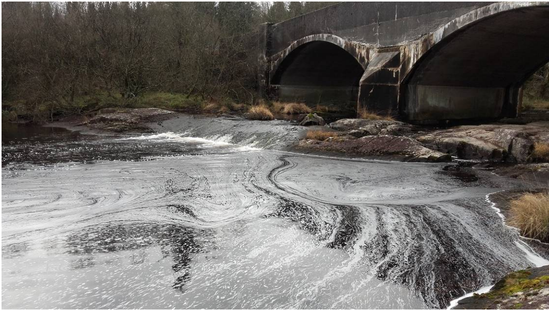
Figure 14: Directly downstream of road bridge at NX 254635 575176, obstruction of upstream migration due to bedrock falls
